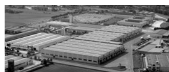
San Giovanni al Natisone (Udine, Italy) Assemblaggio tavoli e sedie, magazzino Tables and chairs assembly lines and warehouse 40.000 sqm
