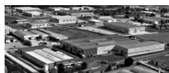
Manzano (Udine, Italy) Assemblaggio sedie, verniciatura e magazzino Chairs assembly lines, varnishing areas and warehouse 19.200 sqm
