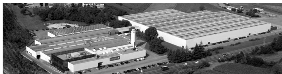
Manzano (Udine, Italy) Sede centrale, R&S, logistica e magazzino / Headquarters, Research & Development, logistics and warehouse 26.000 sqm
